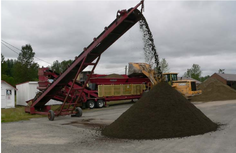
Creation of bioretention soil media/mix (BSM) composed of 60% compost and 40% sand
