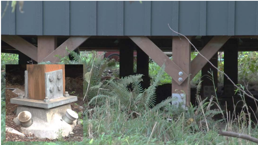
Home built with a PIN foundation system.
