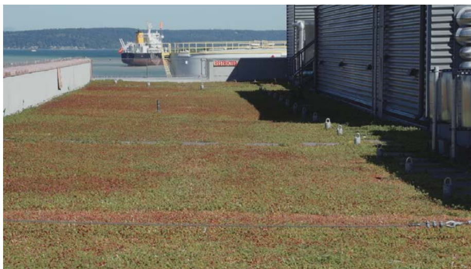
Vegetated roof planted with sedums
