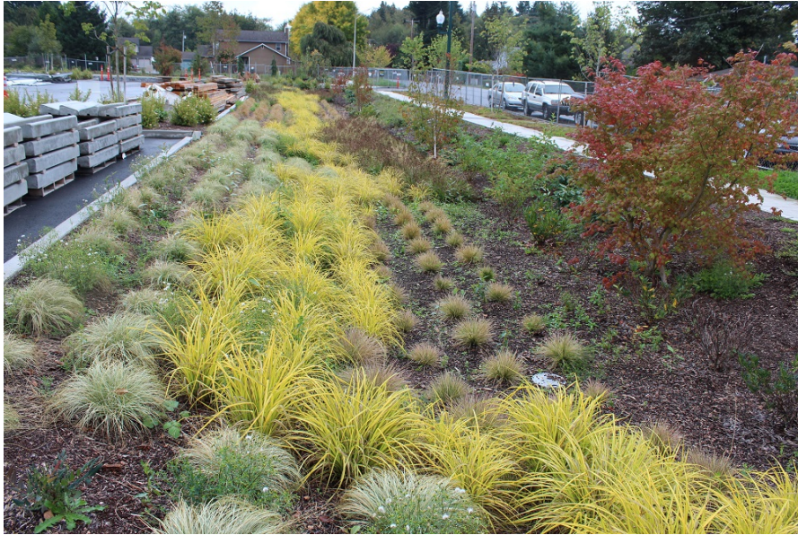
Large bioretention facility in Western Washington
