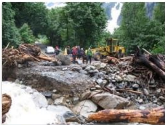
Figure 3. Cascade River Road, August 2013. Heavy rain mobilized river debris clogging a culvert. The road washed out, stranding 70 visitors and their vehicles for 2 days.
