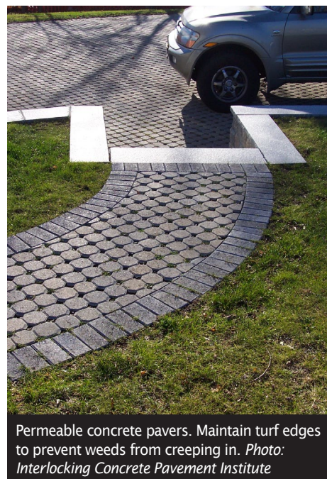
Well-maintained pervious concrete will allow water to soak right in! Photo: Erica Guttman
