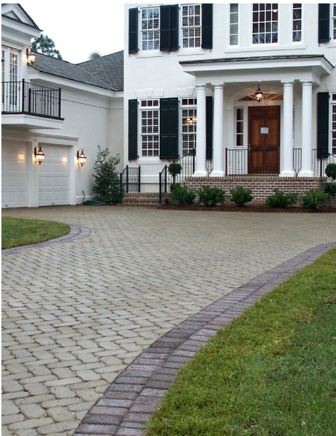
Pervious pavers filter and manage water on site. Photo: Interlocking Concrete Pavement Institute.
