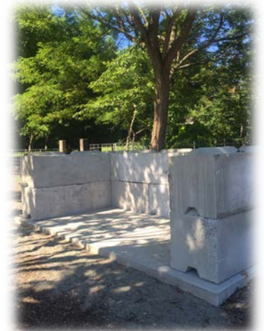
Waste Storage Structure
