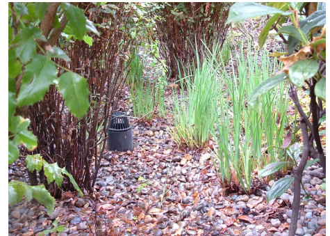
It's important to keep inflows and overflows clear of litter and vegetation. Photo: Erica Guttman
