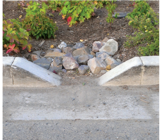
Remove leaves and other debris from rain garden inlets and outlets
