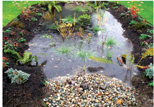
Some rain gardens will pond like this during rain events, others will drain as fast as they fill
