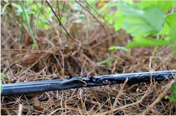
▲ Your monitoring visits should include inspection of irrigation systems, ensuring that no components are damaged so water is being wasted. Irrigation-system leaks that prevent or significantly reduce planned watering rates should be evident by noticing drought stress on the hedgerow's plants. (Photo: Stephen Bramwell)
