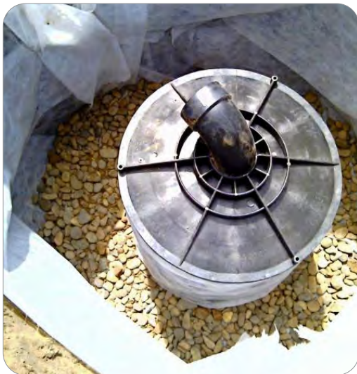
Photo: Eco Plumber, Portland
