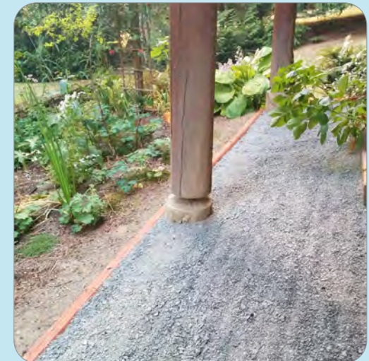
Added drain rock under this deck's drip-line will SLOW runoff and reduce erosion.
