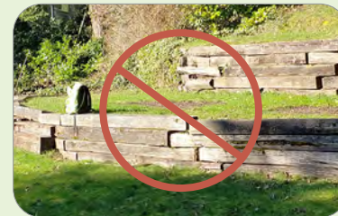
WOOD RETAINING WALLS
