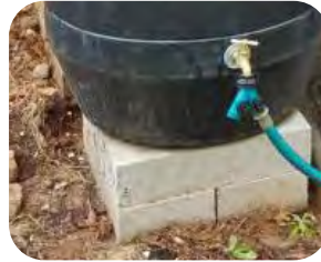
Cinder blocks, laid side-by-side fully support the bottom of the tank(s)
