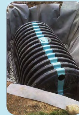
Photo: Earth, Stone & Water
