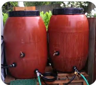
Collect more water by connecting several tanks together.
