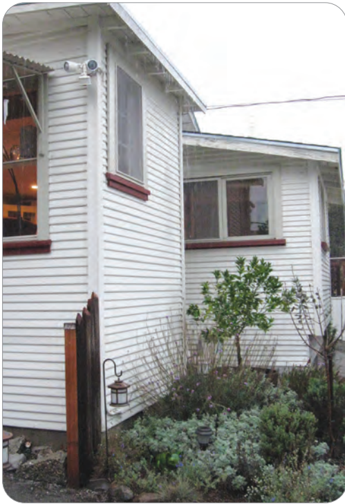
Stable vegetation under your roof's eaves will prevent erosion at your home's foundation.
