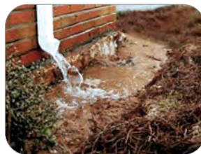
Photo: Northern Virginia Soil and Water Conservation District
