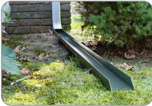
Splashblocks SLOW runoff and carry it away from your home's foundation or crawl space.
