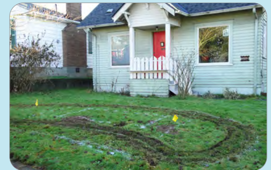
Upon request, utility companies will mark the utility locations on your property using colored flags or spray paint.
