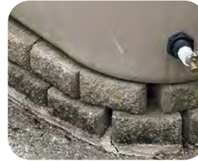
Interlocking bricks surround and retain a bed of packed, crushed rock
