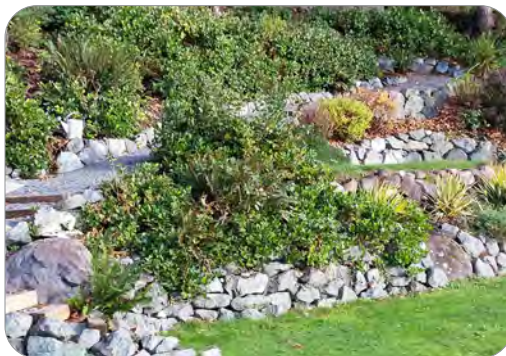
Terraces create relatively level 'steps' on slopes for plantings and landscaping to SLOW rainwater down.
