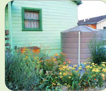
Cisterns come in a range of sizes and can hold 200 to 1,000 gallons or more.
