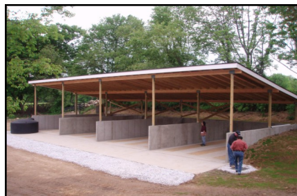
Covered four- section manure storage
