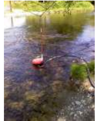
Fence and solar pump installation on Friday Creek, Samish Watershed
